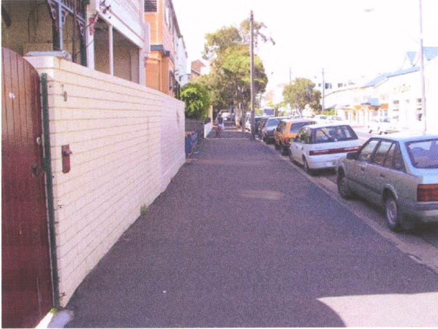
PAVING TYPE 5 – Pittwater Road – Bitumen.
