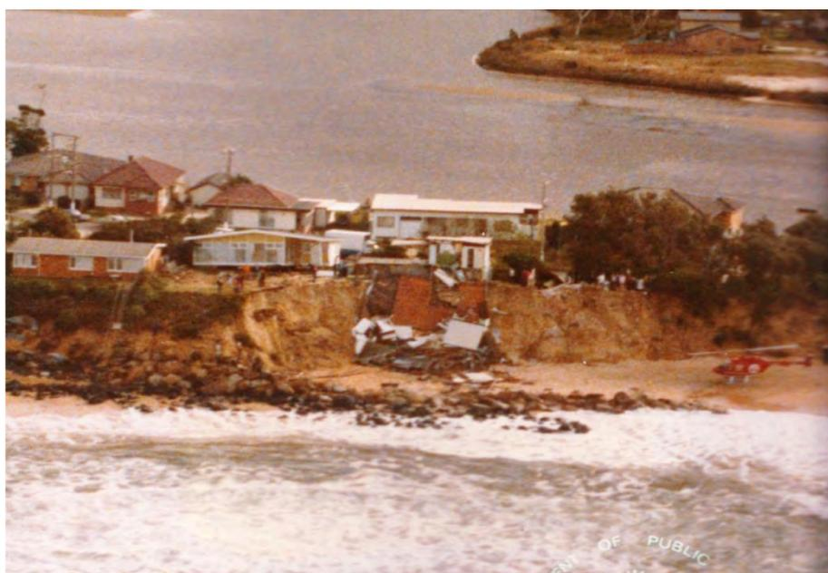
**Figure D18: Erosion landward of revetment at Wamberal Beach in June 1978**
