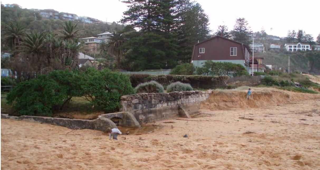
**Figure A11: Vertical seawall at 21 Bilgola Avenue, partially exposed after storms on 21 July 2007**
