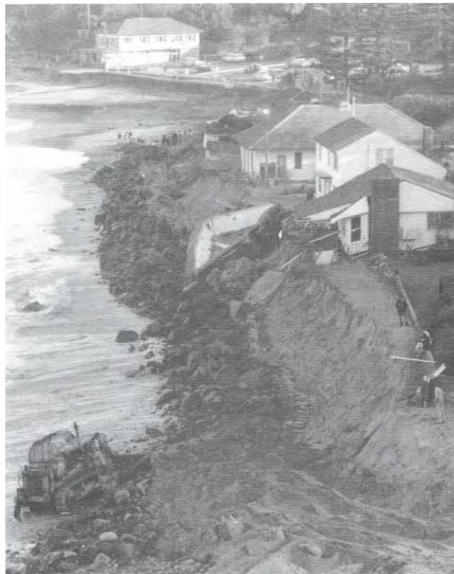
**Figure A9: View looking south of storm damage and rock protection at Bilgola Beach on 11 June 1974 (from PWD, 1985)**
