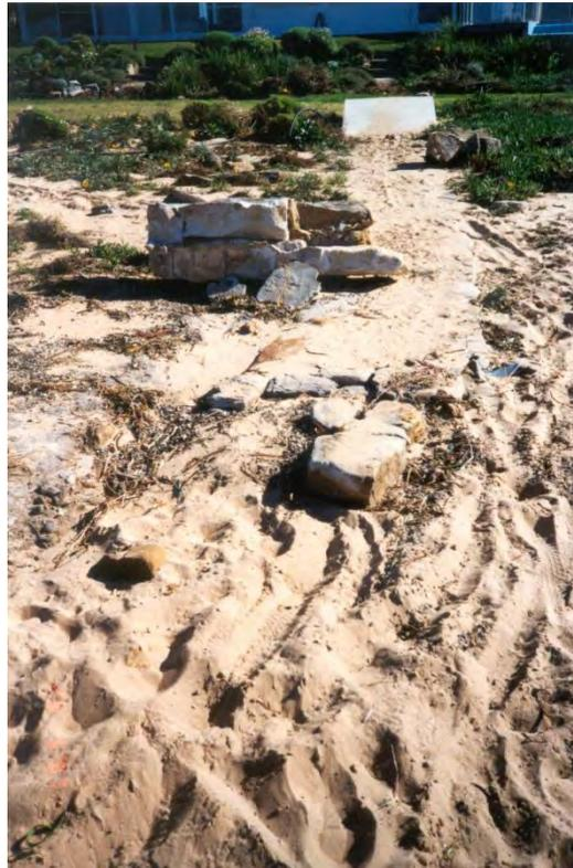
**Figure A13: Evidence of damage caused to vertical seawall seaward of subject property during May 1997 storm, with blocks carried landward**
