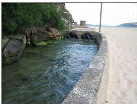
Low-flow pipes at channel entrance
