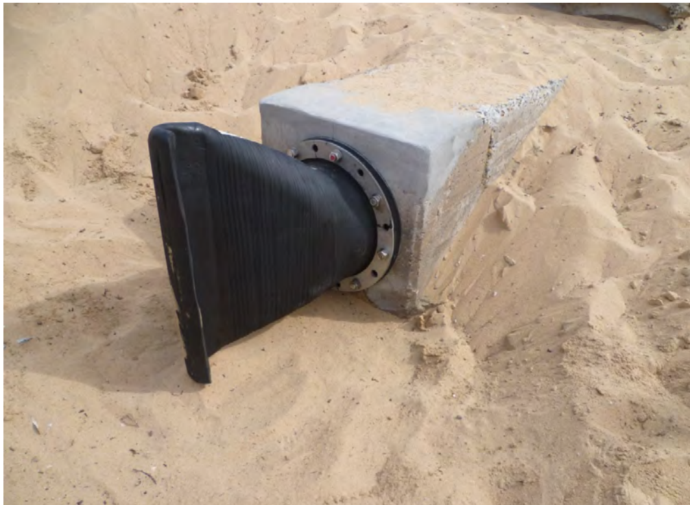
Figure G14: Tideflex 'duckbill' check valve fitted to Frazer Street outlet, 22 August 2013
