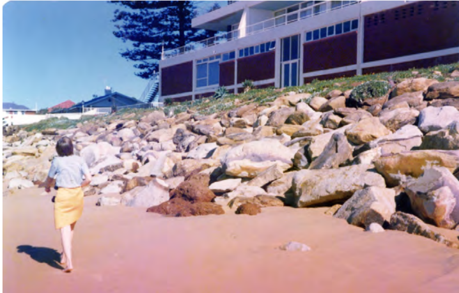
Figure C4: Closer view of rock protection visible at “Flight Deck” sometime between 1969 and 1974 (courtesy of Mr Don Champion)
