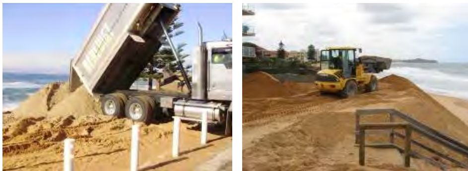
Figure I4: Bogie tipper truck depositing sand (left), and being spread by machinery (right) at Collaroy-Narrabeen Beach
