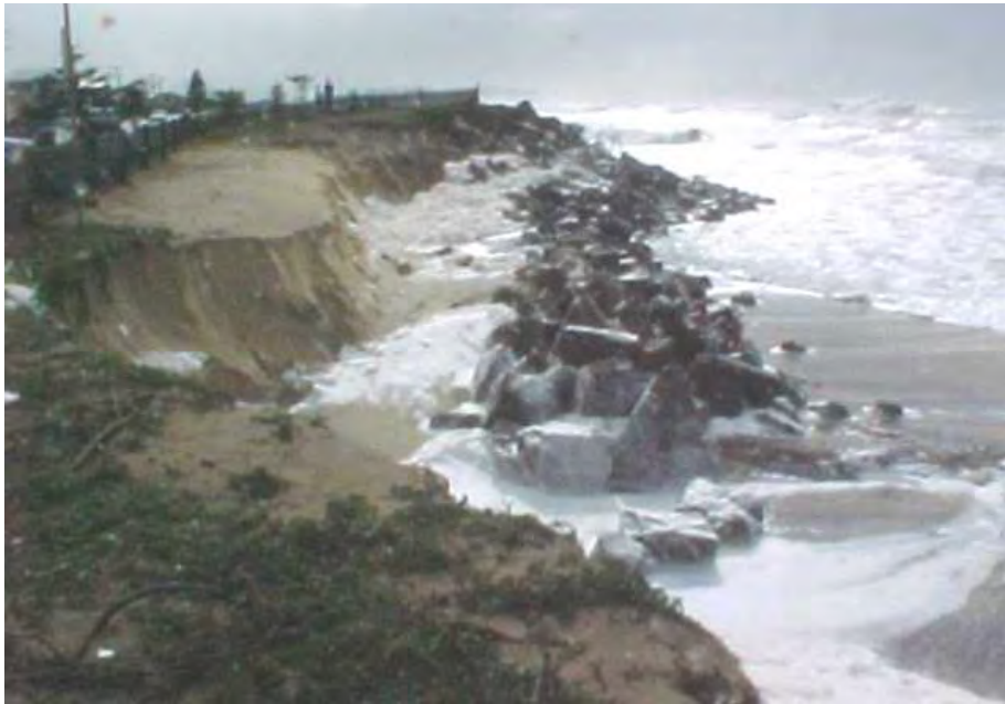
Figure L8: Erosion landward of revetment at Stockton Beach in July 1999
