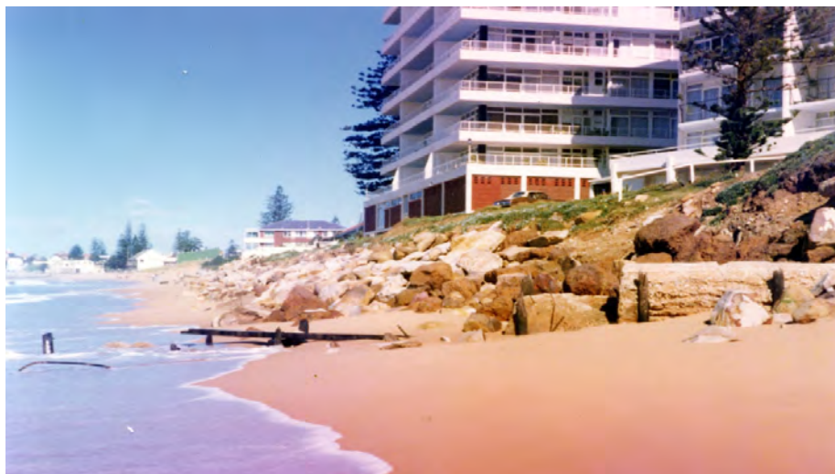
Figure C3: Rock protection visible at “Flight Deck” (left) and “Shipmates” (right) sometime between 1969 and 1974 (courtesy of Mr Don Champion)
