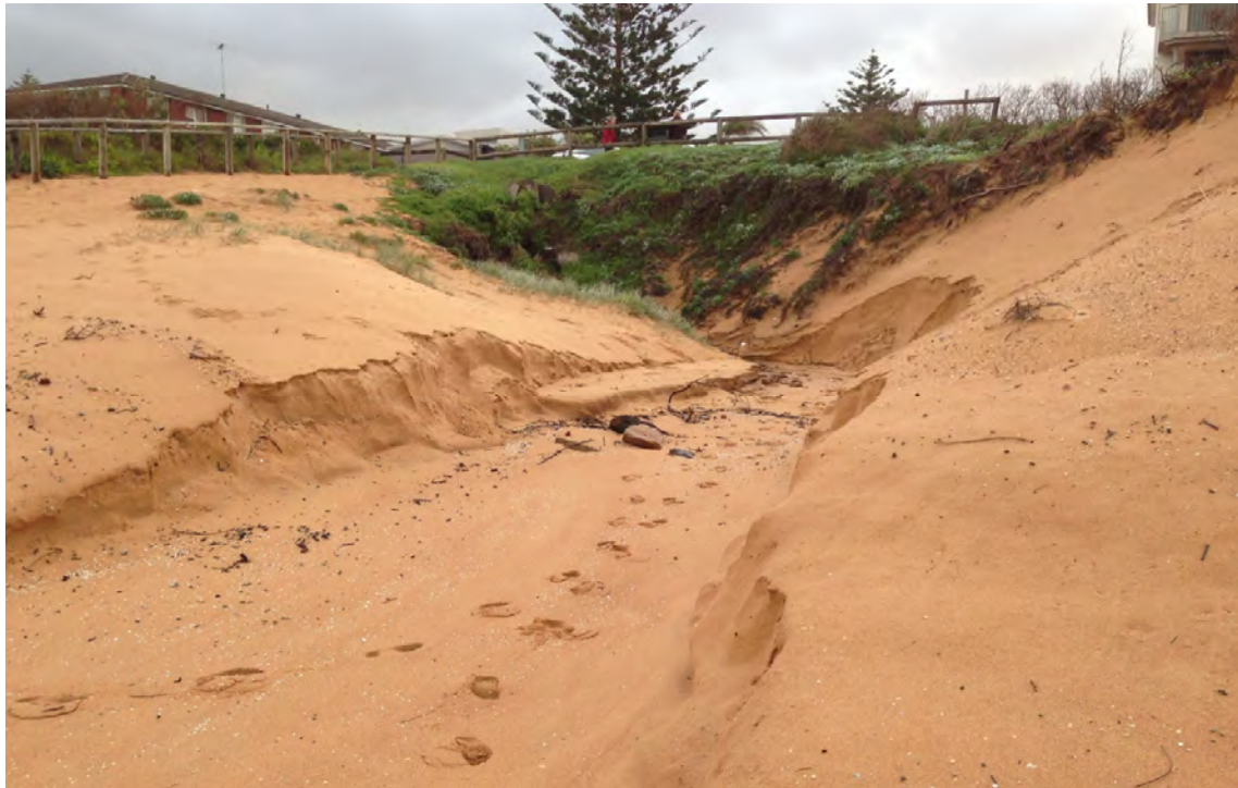
Figure G3: Scour at stormwater outlet near Tourmaline Street at Narrabeen, 20 April 2013
