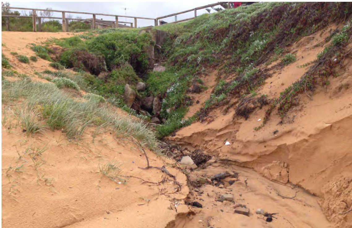
Figure G4: Closer view of stormwater outlet and scour near Tourmaline Street, 20 April 2013
