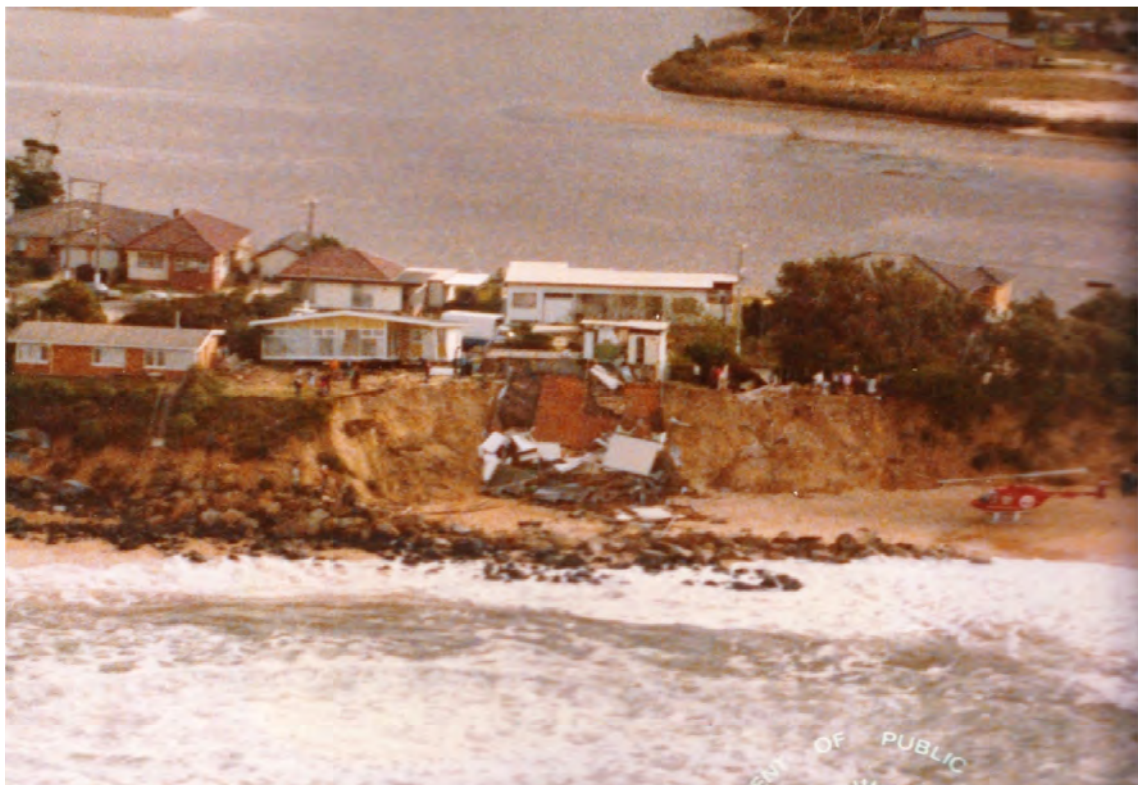
Figure L9: Erosion landward of revetment at Wamberal Beach in June 1978
