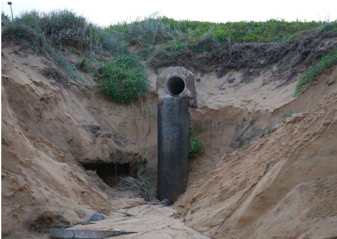
Figure G2: Stormwater outlet near car park south of Malcolm Street after erosion, 25 June 2013
