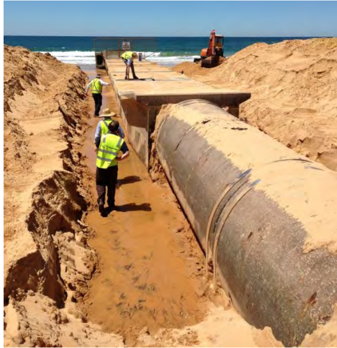
Figure G17: Excavation surrounding the Collaroy Street outfall as part of investigations for proposed reconstruction works, 14 November 2013
