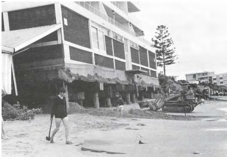
Figure C2: Exposure of “Flight Deck” foundations as a result of 1967 storms (from PWD, 1985)
