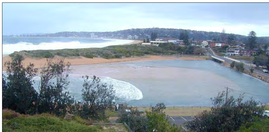
Figure 6-5 Waves overtopping into Narrabeen Lagoon
