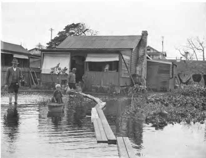
Flooding in Narrabeen, April 1927
