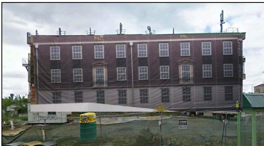
Figure 6 – Building Wrap Concept – significant scaffold is required to attach the mesh screening.
