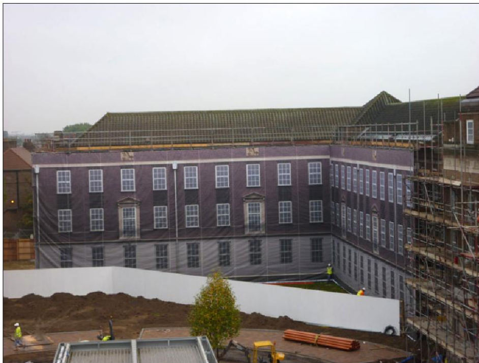
Figure 3 & 4. Examples of building 'Skinning' – mesh (top) and vinyl (bottom)
