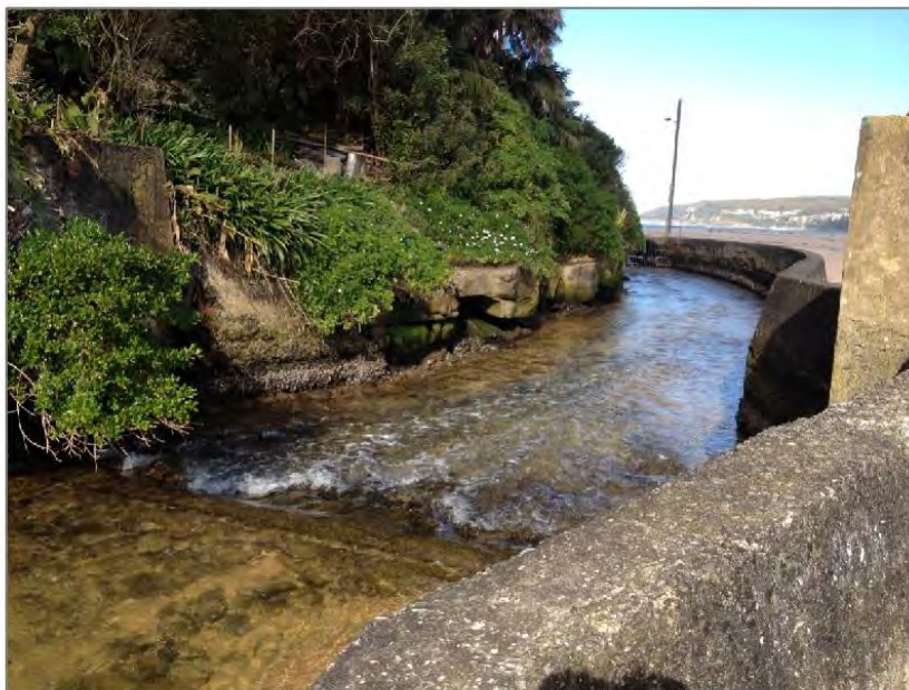
Figure 6-4 Manly Lagoon concrete entrance channel
