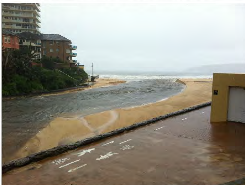
Figure 6-5 Scoured entrance during March 2011 event (Source: MHL)
