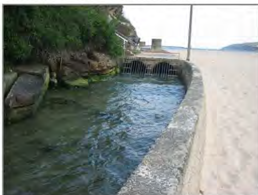
Low-flow pipes at channel entrance
