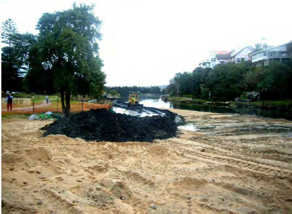
Figure 14: Shot of the bulldozer pushing sediment up into a pile on the shore, June 2006.
