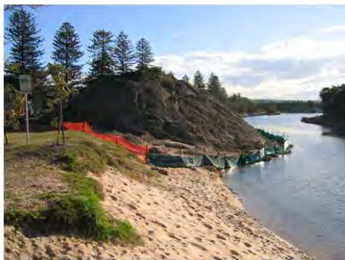
Figure 6: After the marine sand has been dredged, August 2006, showing the sand stockpile on the shore. Discoloration is due to estuarine fines.
