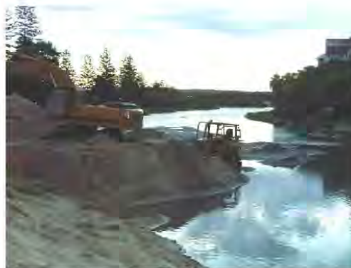
Figure 8: During the entrance dredging. Dredging is done through a bulldozer pushing sand up against the shore then piled up by an excavator.
