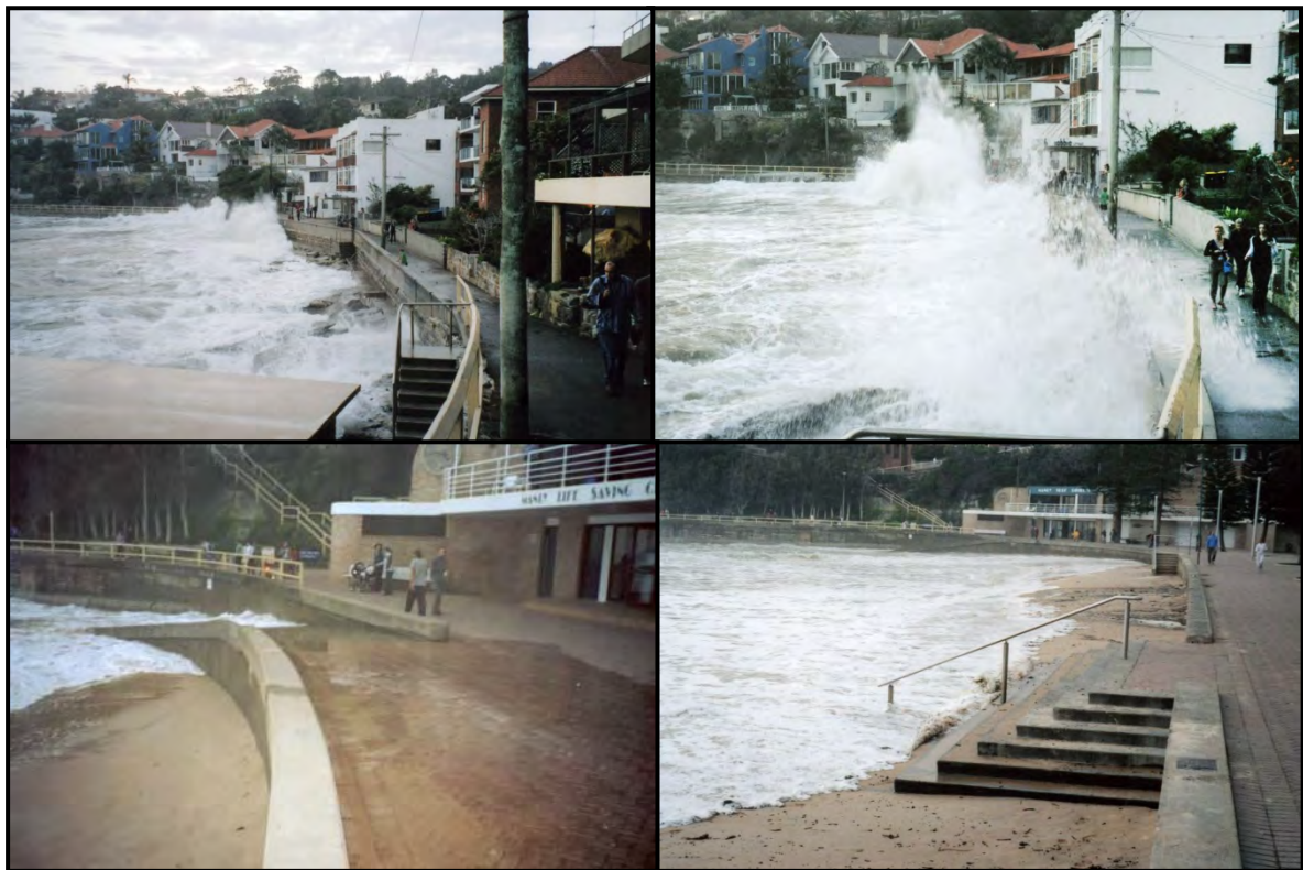
Figure 4.6 Top Photos Wave Overtopping at Fairy Bower; Bottom Photos Wave Runup at Manly LSC Boat Ramp and Manly Beach Stairs at Victoria Pde (26/06/2003 Photos James Carley, WRL)
