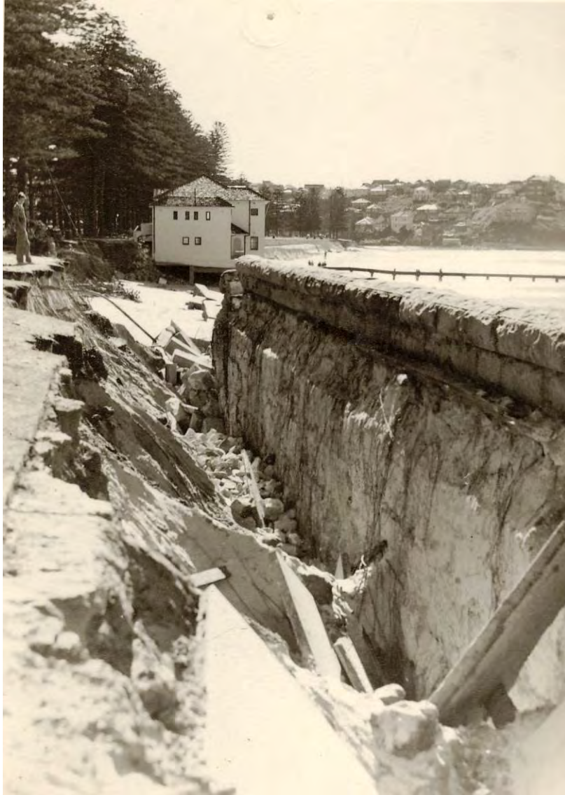
Figure 5.2 North Steyne Collapsed Seawall 27/06/1950
