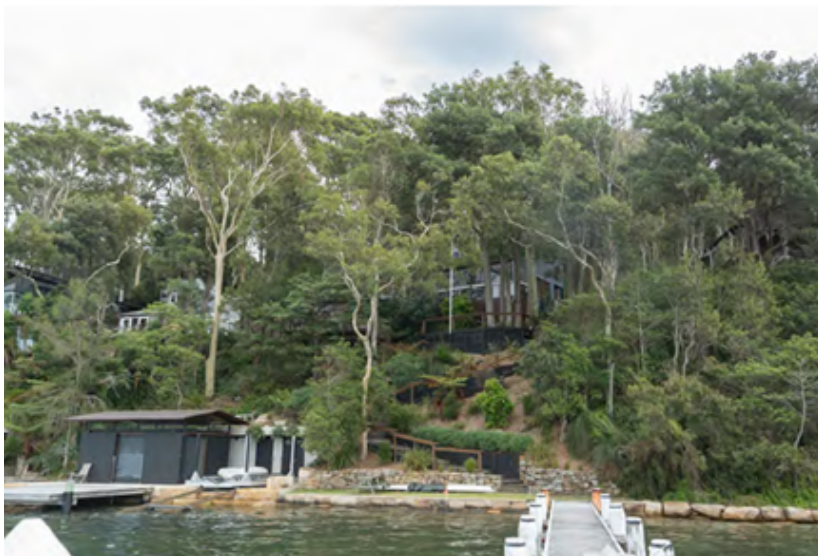
Figure 3 Subject site as viewed from the waterway
