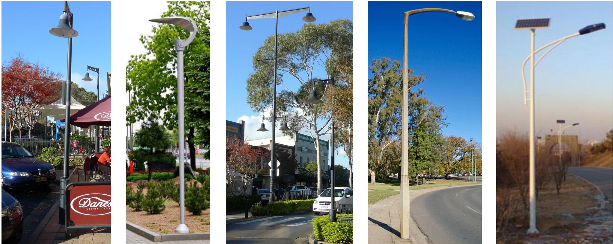
STREET LIGHT - TRADITIONAL OR MODERN WITH LED SOLAR LIGHT
