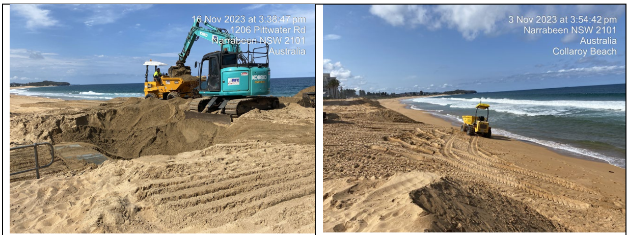
Figure 3-6 View of sand placement on Collaroy-Narrabeen Beach (source: RARE Environmental)
