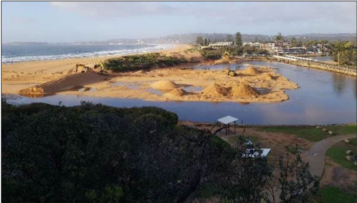
Figure 3-3 View of previous entrance clearance works – traditional excavation methodology (source: RHDHV, 2022)
