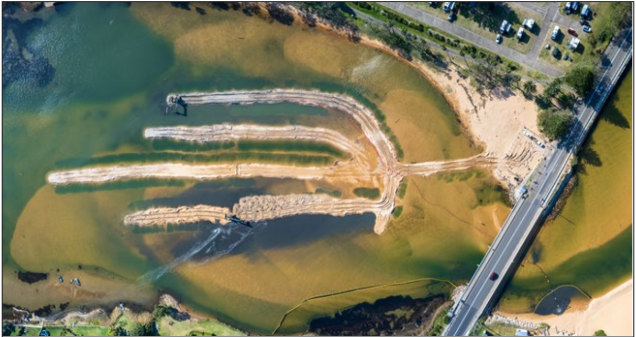
Figure 3-5 View of entrance clearance works – excavator mounted dredge (source: Northern Beaches Council)
