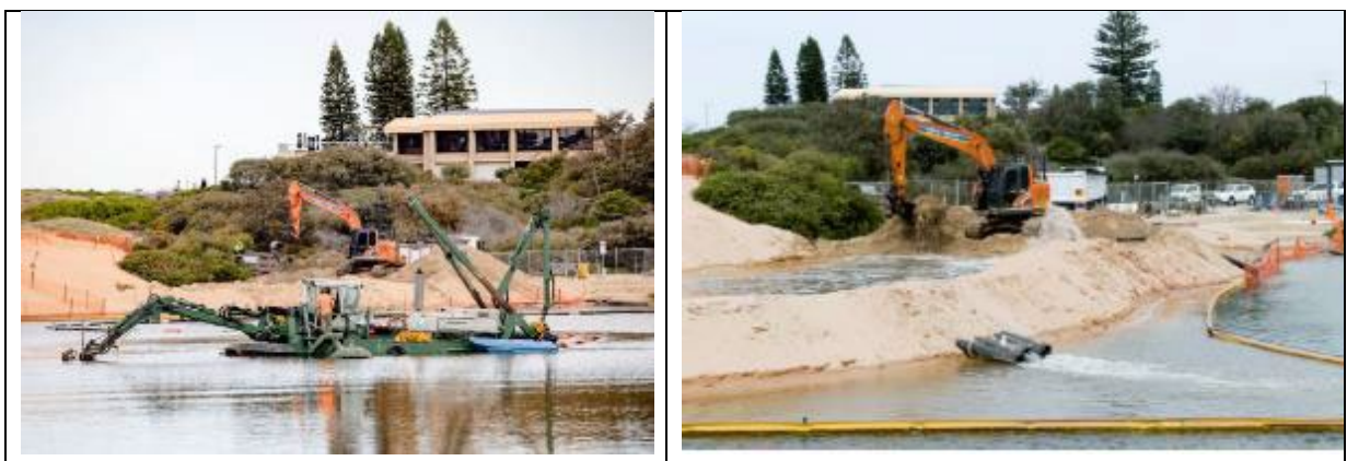
Figure 3-4 View of entrance clearance works – cutter suction dredge methodology (source: SCS, 2022)
