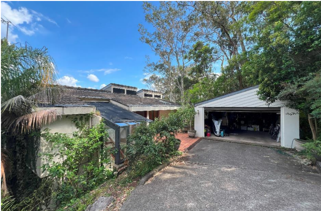
Figure 9 Facing northwest within the subject site towards the dwelling and detached garage. Source: CPS site inspection, 19.02.2025.
