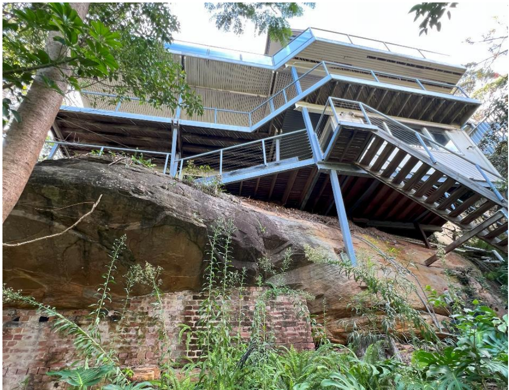
Figure 11 Looking up at the rear of the dwelling and rock outcrop from the densely vegetated rear yard. Source: CPS site inspection, 19.02.2025.
