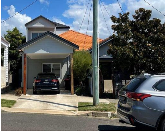
Figure 7 – existing street frontage showing the existing gables and hip roof forms
