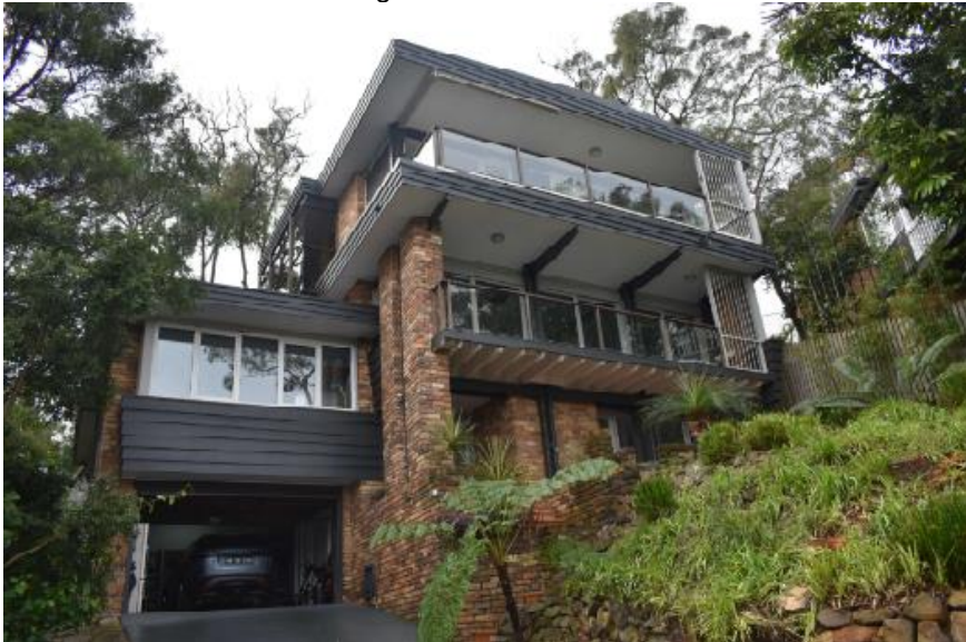
The height and scale of the existing dwelling house establishes a context for the proposed exception
