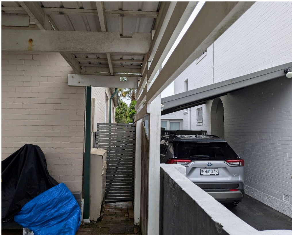
Photo 2: View from subject site of the southern elevation of no. 35 Quinton Road showing the windows that will impacted by the proposed development.
