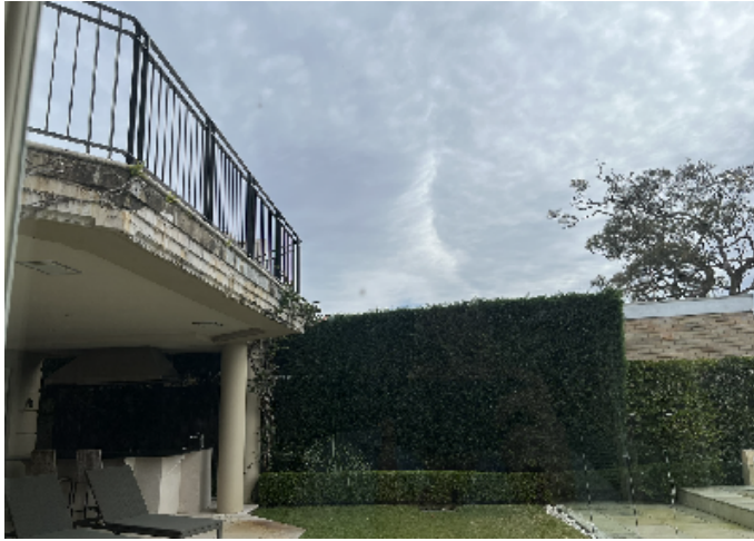
Photo 1 - Ground floor terrace
