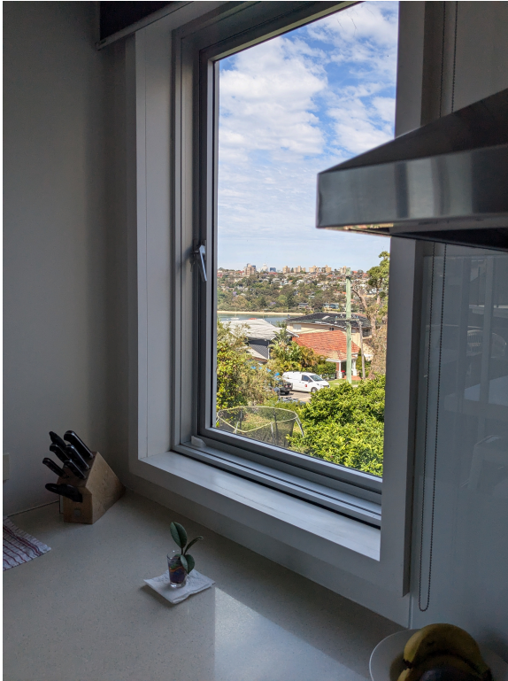
Photo 9: View from west facing kitchen window in standing position - October 2024.
