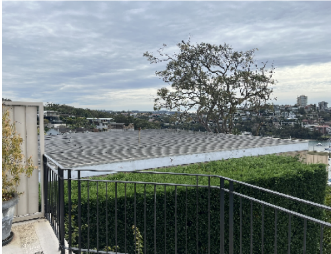
Photo 3 - First floor terrace
