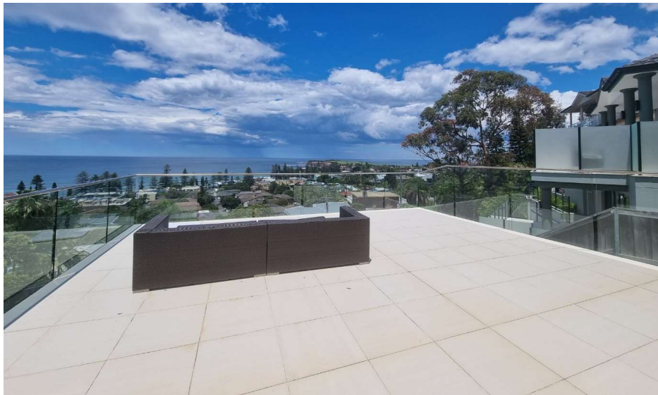
Existing Roof Terrace, 11 Graylind Close
