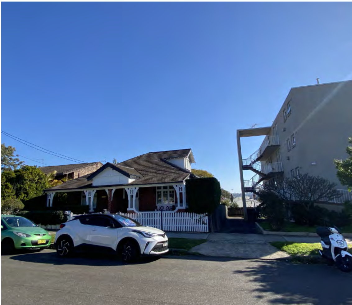
Figure 2 - Subject site (left) and adjoining property to the north (15 Crescent Street) (right) to demonstrate neighbouring scale of development and existing roof form at the subject site, behind
