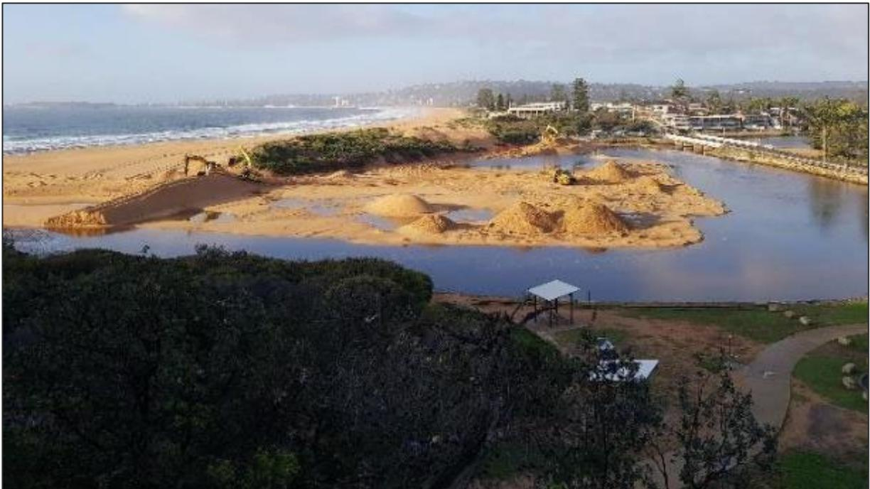
**Figure 3-2: Entrance clearance works – traditional excavation methodology (source: RHDHV, 2022)**
