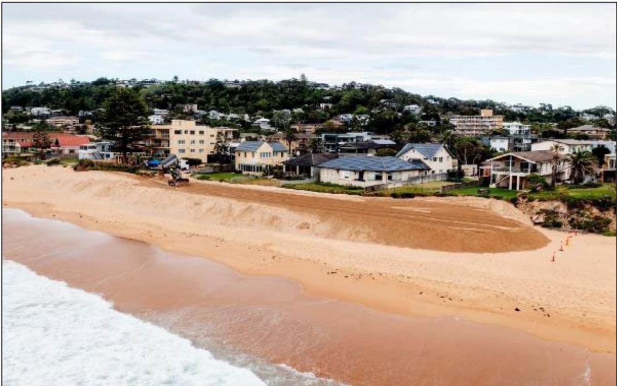
Figure 3-4: 2021 entrance clearance works – dumping sand on Collaroy-Narrabeen Beach (source: SCS, 2022)
