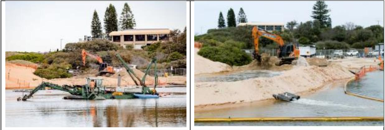
Figure 3-3: 2021 entrance clearance works – cutter pump dredging methodology (source: SCS, 2022)
