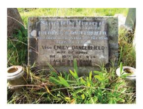
Sometimes black plastic filler is used in place of lead lettering, but it generally does not last well
