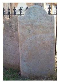
Acid cleaning of marble almost always causes both physical and aesthetic problems
