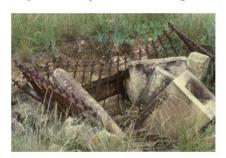
Generally hidden until it happens, the inward collapse of the underground walls of a vault can be disastrous
