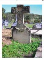
Allowing soil build-up can introduce dampness, which starts the process of surface deterioration
