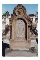
The dampness problem is especially acute if the surface is prevented from washing by rain, as here by a hood moulding in the original design
