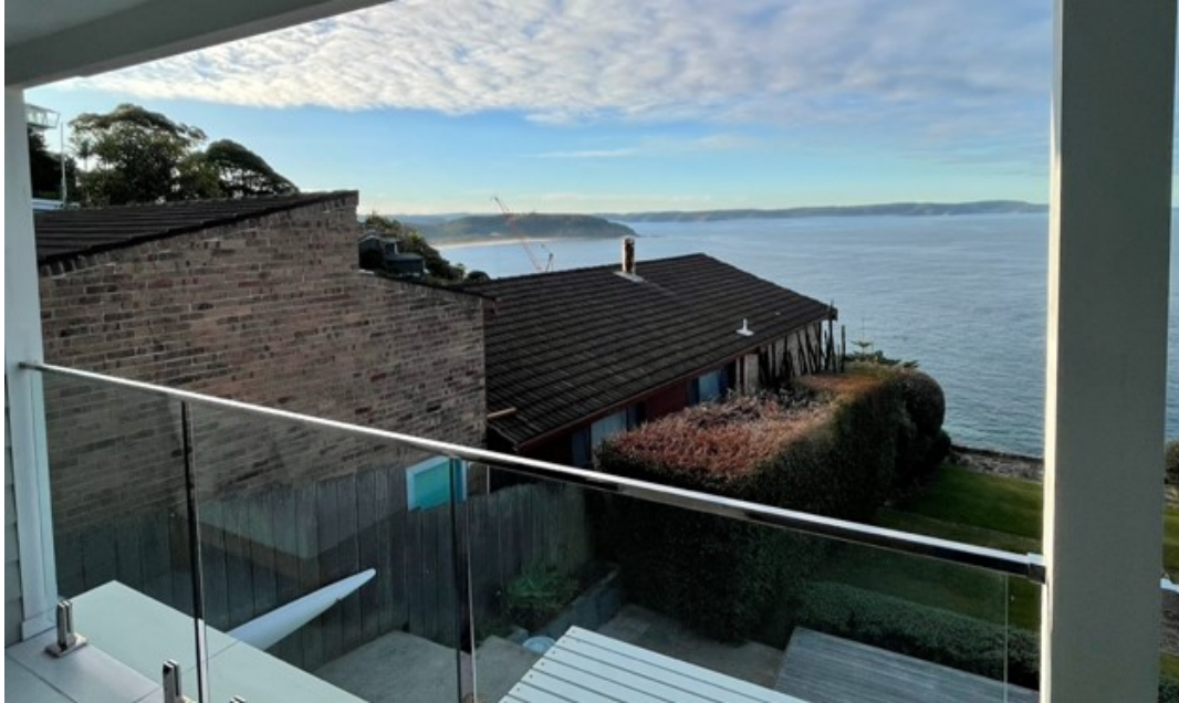
Figure 8 - Balcony adjoining kitchen, photo provided by owner 14 Norma Road, standing position looking north-east.
