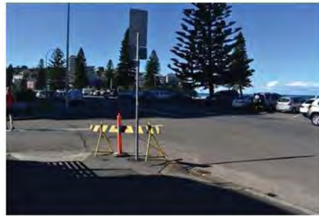
Inappropriately constructed kerb ramp on North Steyne near Ceramic Lane opposite beach – no pedestrian crossing there
