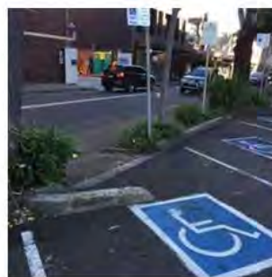
Lack of marked continuous accessible pathway from the car parking to the library or the surrounding area; inappropriately designed parking bay with obstacles
