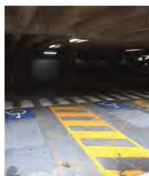
Insufficient lighting at accessible parking area, Ground Level
