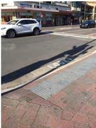
TGS inside the kerb ramp at Manly Wharf
