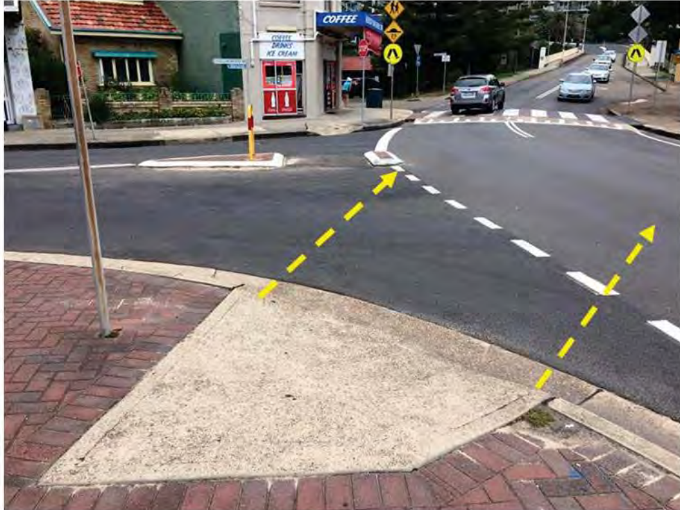
Figure 4.6: North Steyne - Unaligned Kerb Ramp
