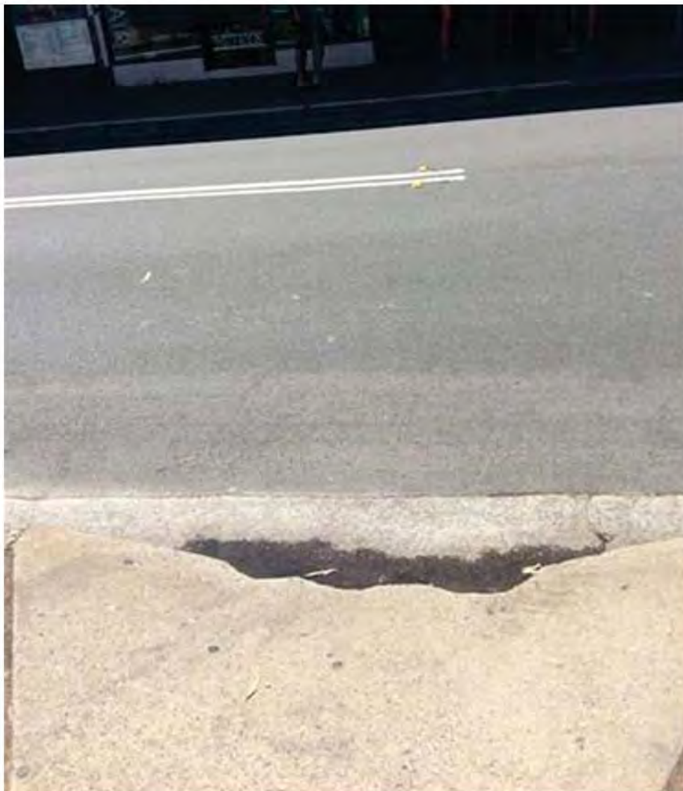
Figure 4.5: Whistler Street - Unconnected Kerb Ramp and Ponding
