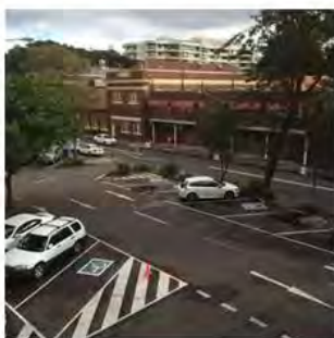
Lack of marked continuous accessible pathway from the car parking to the library or the surrounding area; inappropriately designed parking bay with obstacles
