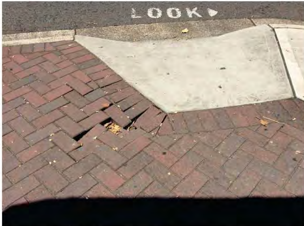
Figure 4.4: Darley Road - Missing and Damaged Pavers near Kerb Ramp
