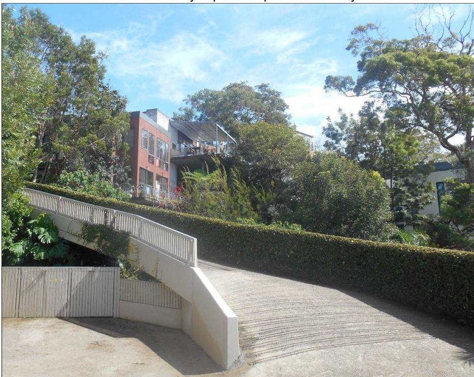
Image: Adjacent dwelling to northwest also overlooks site across driveway area.
