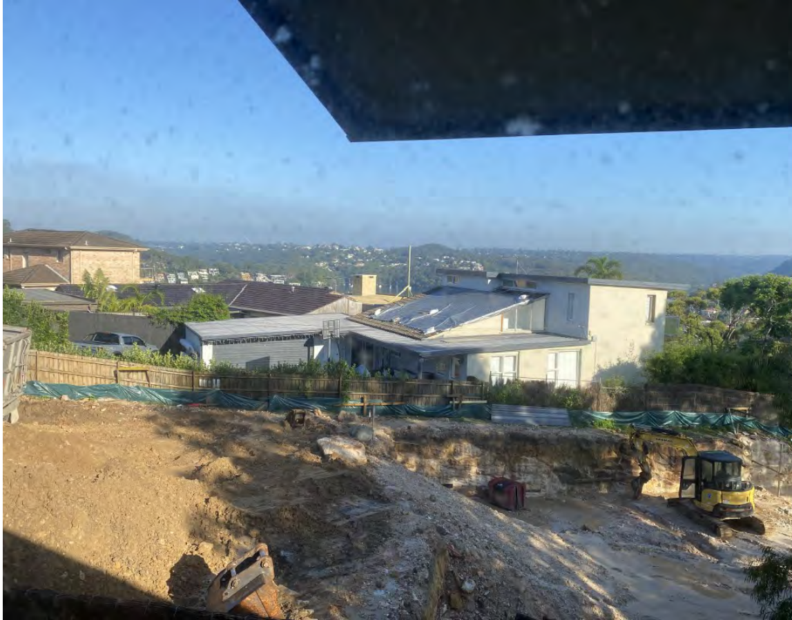
Figure 4 - Looking north-west from bedroom window, upper floor, standing position.
