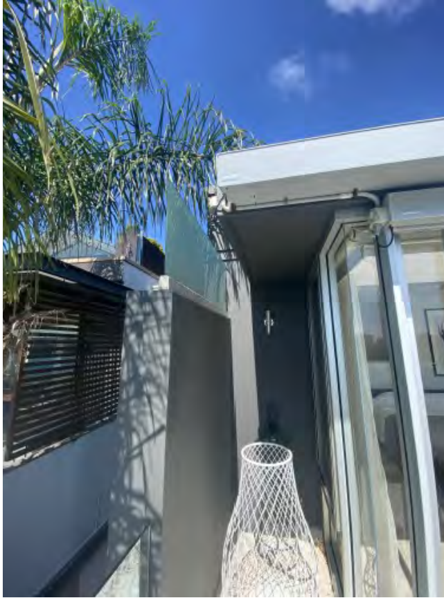
Figure 7 - Corners of balcony on the eastern balconies to be in-filled.
