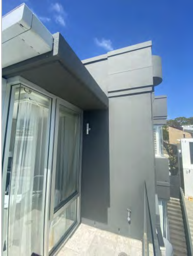
Figure 1 - Corner of balcony on the north-eastern corner to be in-filled.
