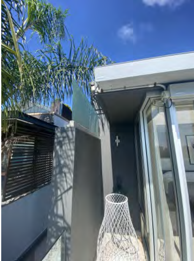
Figure 2- Corner of balcony to be in-filled on the south-western corner. Note - that the wall southern wall is already 3/4 of the height of the balcony.
