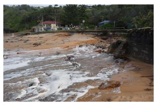
Figure 20: View of scour at northern end of Bilgola SLSC seawall and adjacent to Bilgola Creek and Bilgola Kiosk channel
