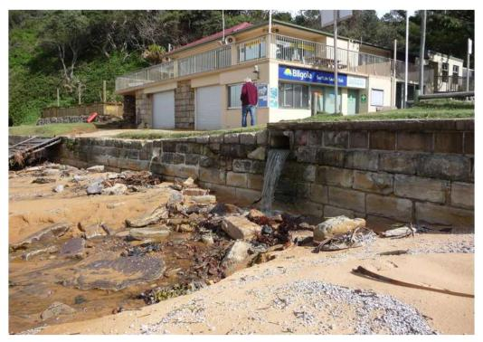
Figure 21: Scour at Bilgola SLSC stormwater outlets
