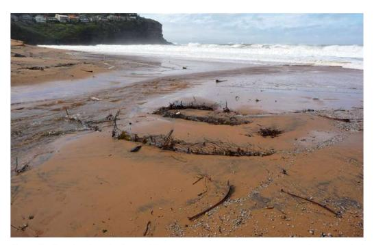
Figure 15: Deteriorating wire from gabion basket or reno mattress scour protection seaward of Bilgola Creek
