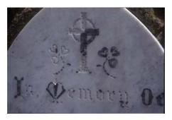
Poorly executed lead lettering can be saved if an expert mason re-fixes the lead before extensive failure
