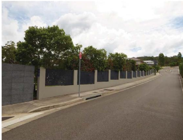
Figure 28 View west along Fazzolari Avenue showing Gate 3 at far left and the recent northern boundary fence of rendered masonry dwarf wall and piers with metal palisade panels. (Photo: Chris Betteridge, 28 January 2016)
