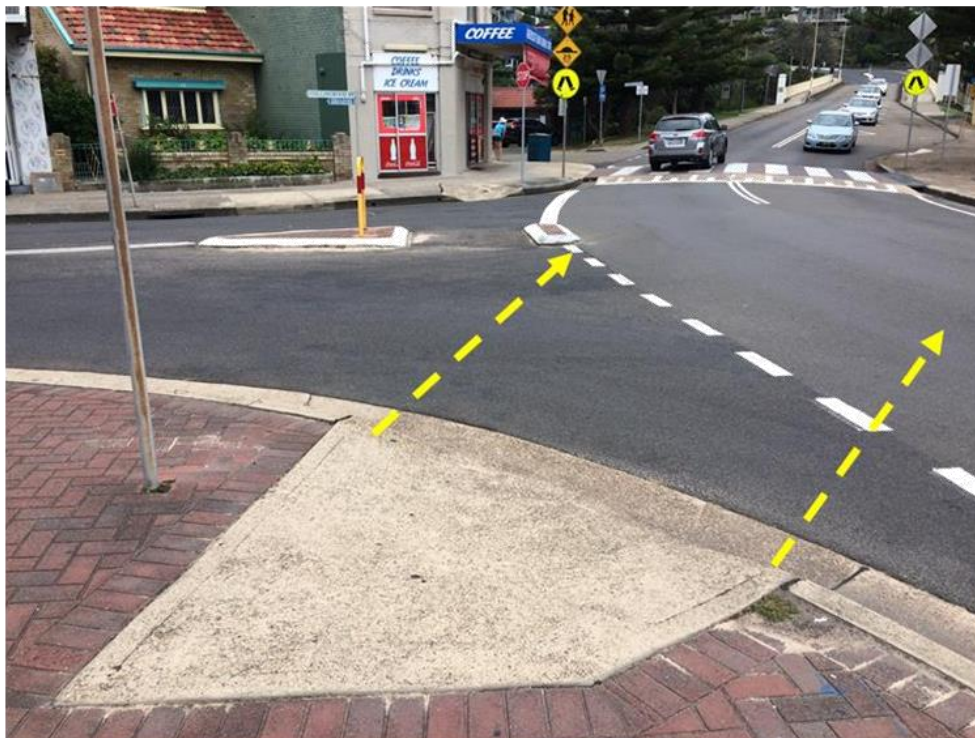
Figure 4.6: North Steyne - Unaligned Kerb Ramp
