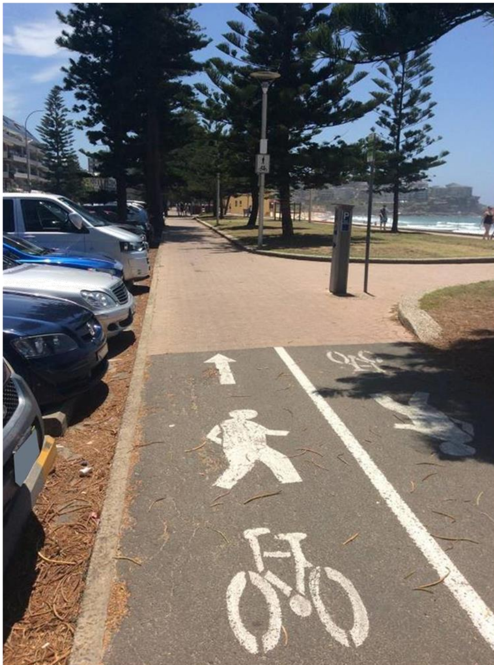
Figure 6.23: Manly Foreshore Shared Path Missing Linemarking
