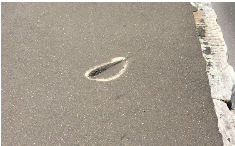
Figure 4.3: North Steyne - Hole in Pavement
