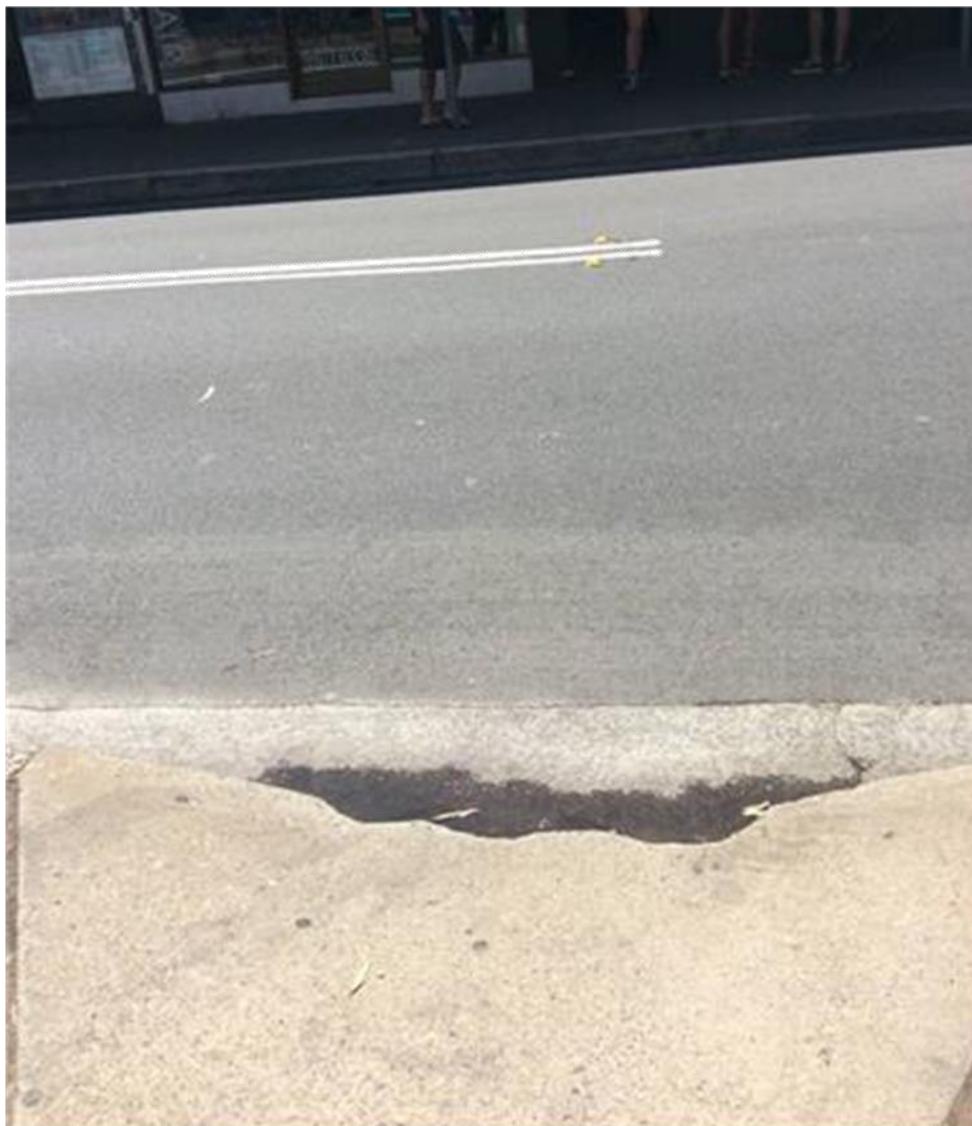
Figure 4.5: Whistler Street - Unconnected Kerb Ramp and Ponding
