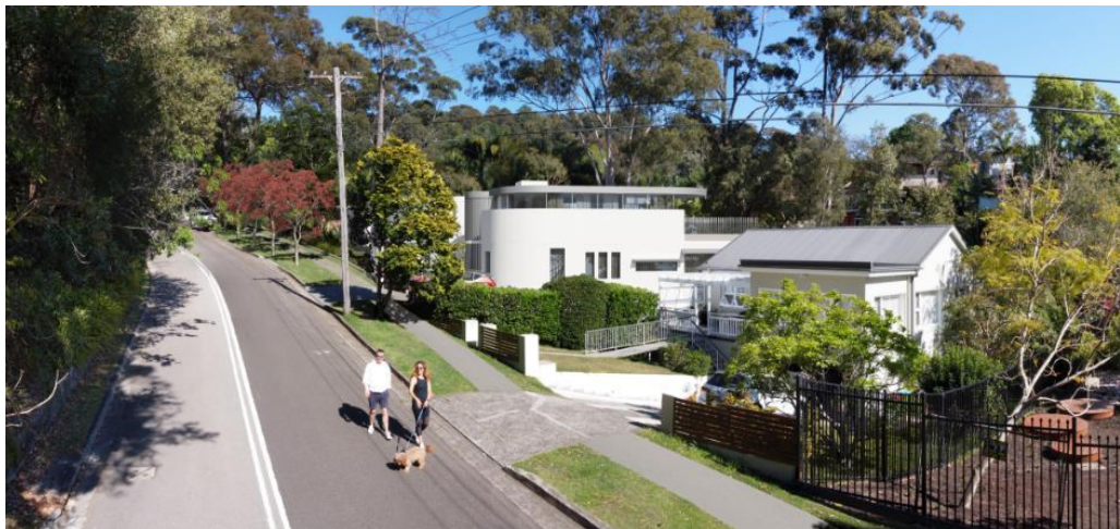
Figure 4 - Photomontage looking up Loquat Valley Road alignment past subject property
