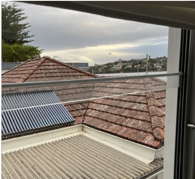
Photo 10- View looking south from the first floor hallway
