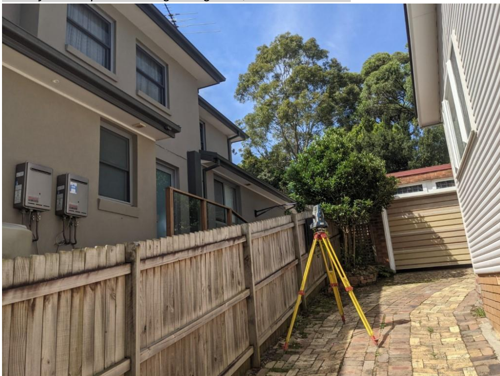
Image 9: Existing slope of the subject property and the adjoining property at 18 Alameda Way.
