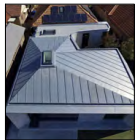
METAL ROOF SHEETING -STANDING SEAM
