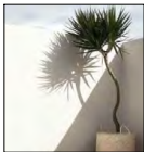
MASONRY WALL -RENDERED WHITE
