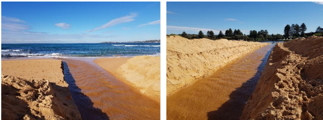
Figure 2-15: Mechanical opening of the lagoon entrance (4 June 2021)
