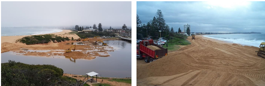
Figure 5-1: Excavators removing the entrance shoals (left), Unloading and regrading of sand for beach replenishment (right)
