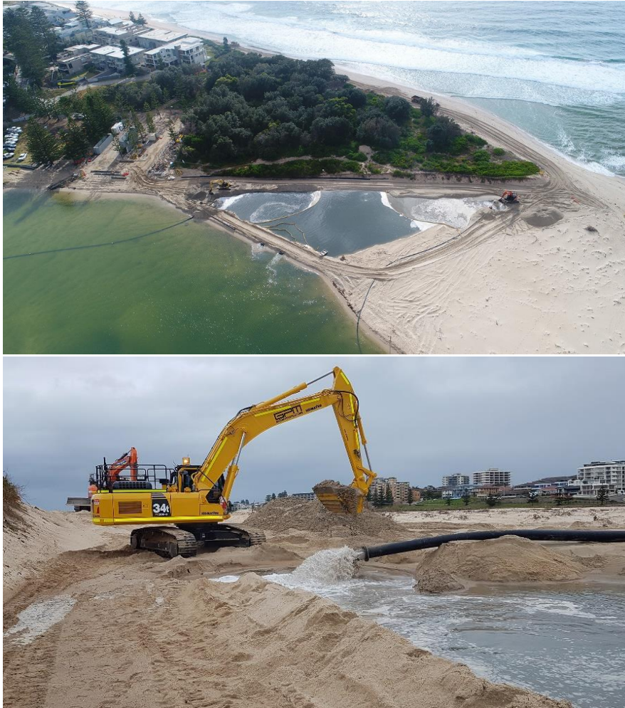
Figure 6-6: Management of sand slurry discharge within a bunded beach area at The Entrance, Central Coast
