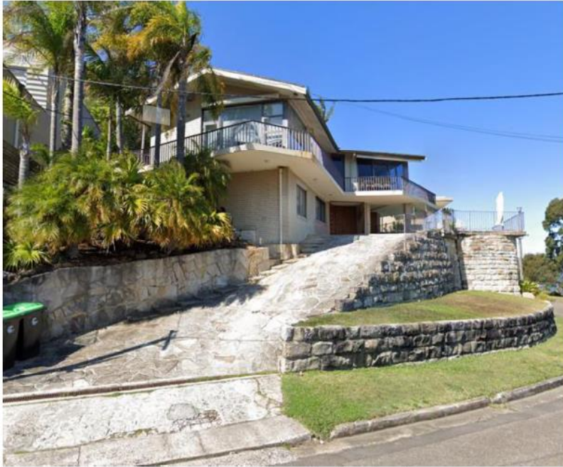
Figure 3: Subject site as viewed from Castle Circuit
