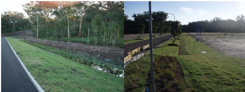
Figure 7-5 Grassed roadside filter strips
