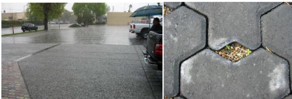
Figure 7-4 Pervious concrete (LHS) and permeable pavers (RHS)
