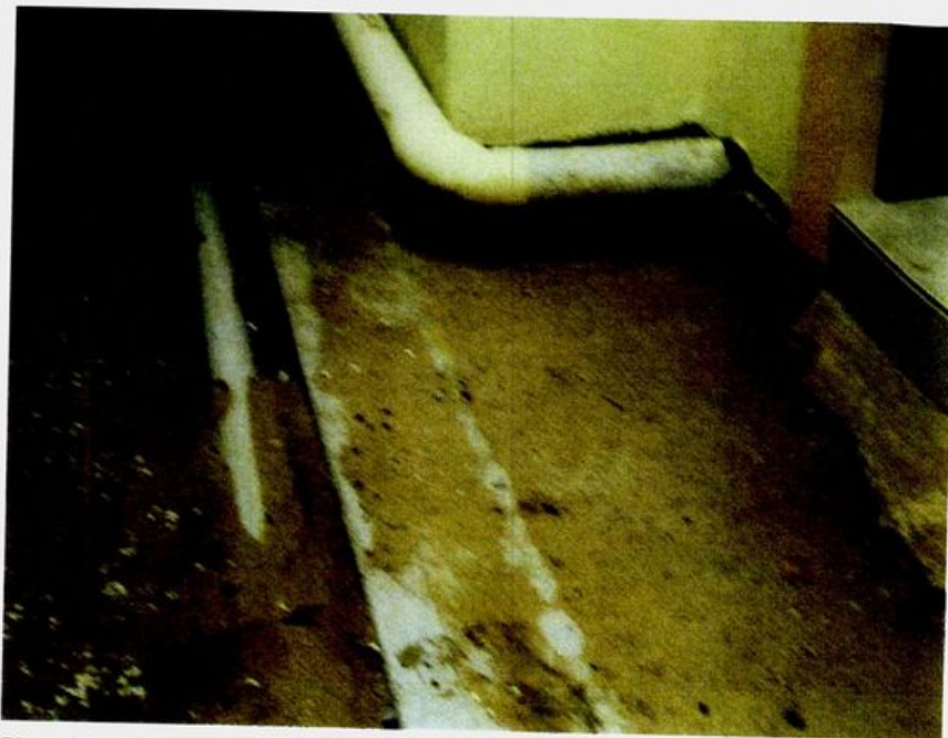
Photo 10 - Slab edge eastern wall at laundry door showing original slab under new slab and showing sewer line penetrating slab edge approx 30 mm above rebate (i.e. within 60 mm of the top of slab. JHC Drawing No. 1 indicates return rib at this location. Maybe line is enclosed at the side of the rib.
