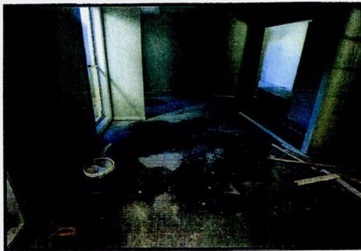
Fig 6 – Result of flood testing within first 30 minutes – water leaking through Main Bathroom floor and Dining Room ceiling directly settling on Dining Room floor.
