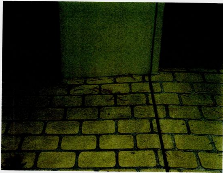
Photo 11 - Eastern side of garage door showing no step in to out and that tiling leading up to front door is above garage floor level.
