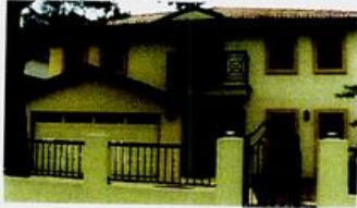
Foamboard type cladding
