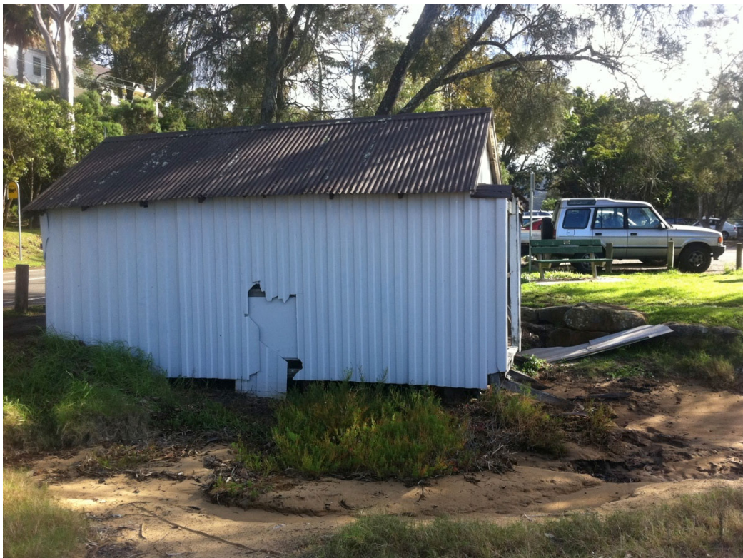
Note erosion from stormwater from road, each end has collapsed and hole in wall
