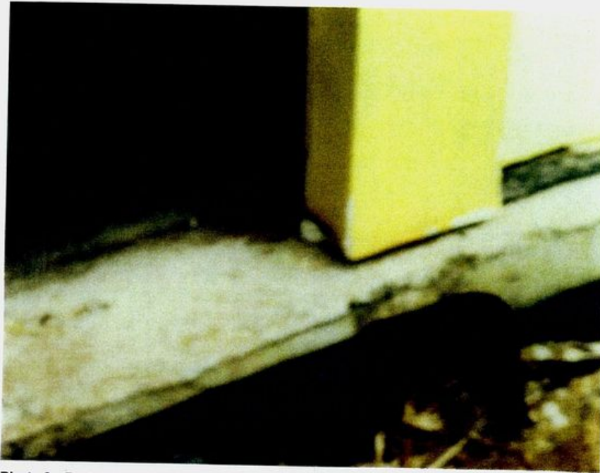
Photo 9 - Part western wall of the rumpus room showing the 1 course edge rebate
