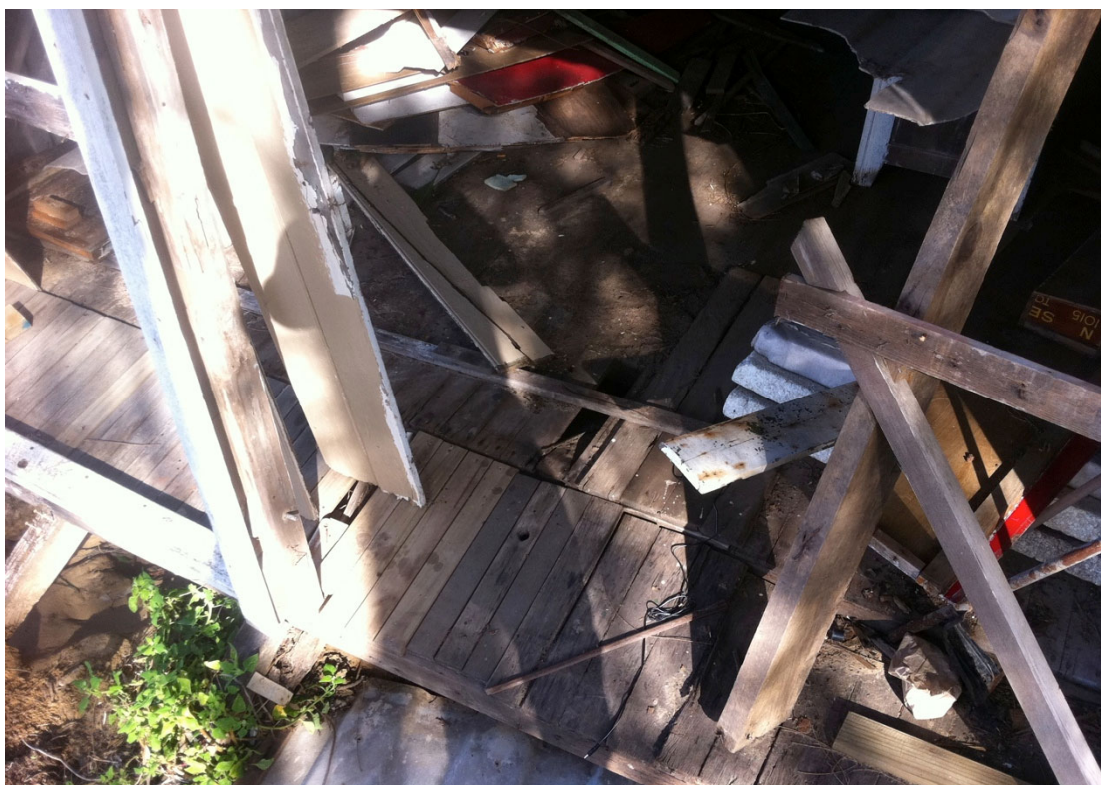
Water front side of boatshed with collapsed flooring joists & floor
