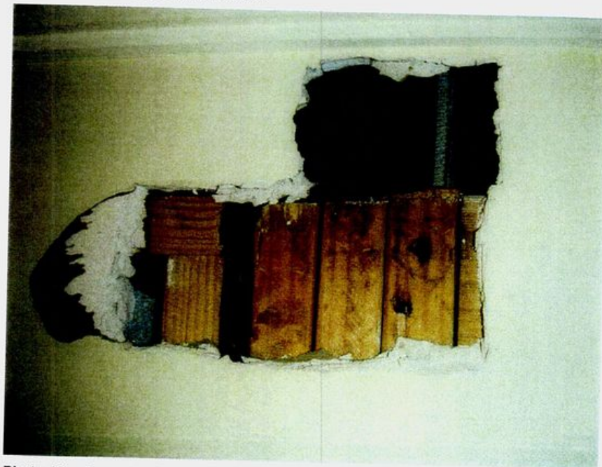
Photo 16 - Support of the beam over the kitchen to meals wall in its south end. Note flange is nearly flush with west face of stud, i.e. beam is about 25 mm eccentric to stud and is not connected to stud.
