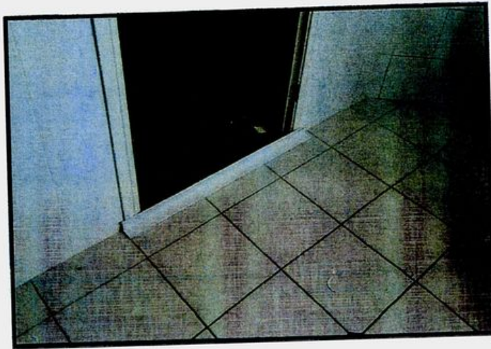
Fig 1 – Preparation of flood testing of first floor bathrooms – see stopper at doorway.
