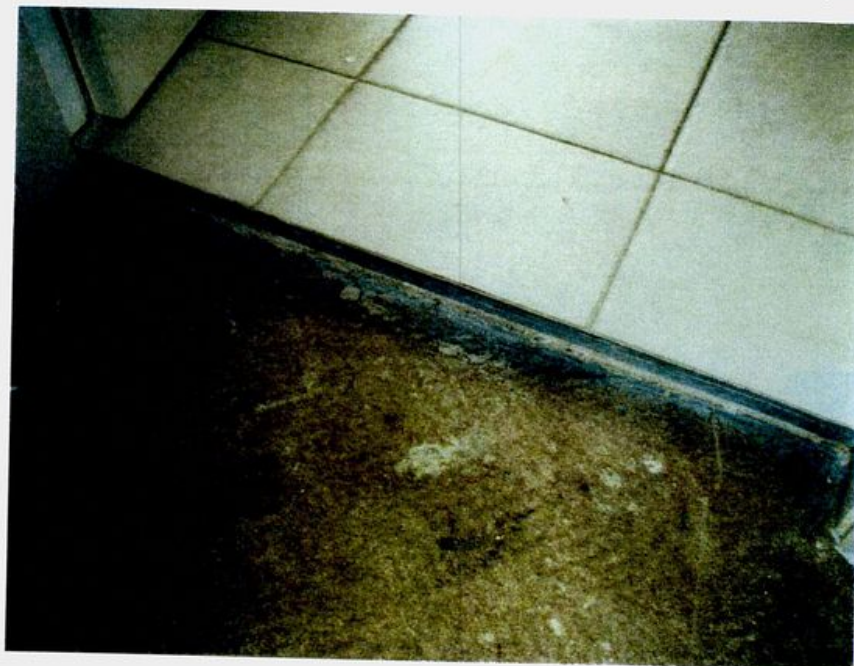
Photo 14 - Bathroom door showing particle board underlying tiles (confirmed from below) and waterproofing extending out onto particle board beyond door, i.e. no indication that membrane was sealed to and turned up an edge angle.
