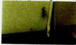
Ground level lowered to expose slab edge.
