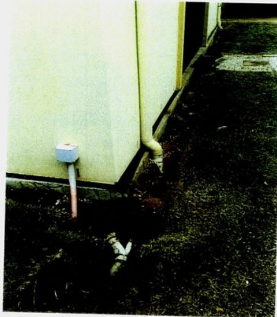
Photo 3 – North west corner of residence (rumpus room) looking south at 90mm dia PVC pipes and main collection pipe.
