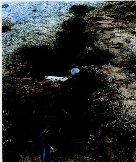
Photo 5 – Rear yard looking at single absorption trench 1.5m long and 90mm dia riser.
