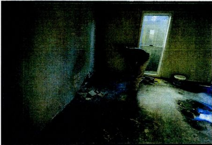
Fig. 10 - Result of flood testing two days after – water ponding in several places of the Dining Room floor.
