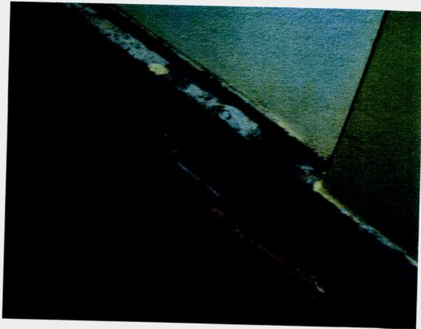
Photo 7 - Slab edge just to the south of Photo 6 where brick course steps and slab edge thickens to 200 mm
