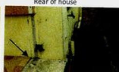
Front and back patios slabs abutting main slab to be removed.
