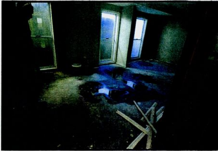
Fig. 10 - Result of flood testing two days after – water ponding in several places of the Dining Room floor.
