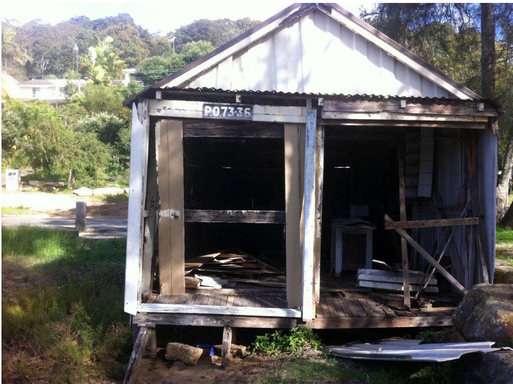
Back of boatshed on the edge of the water showing collapsed floor and piers
