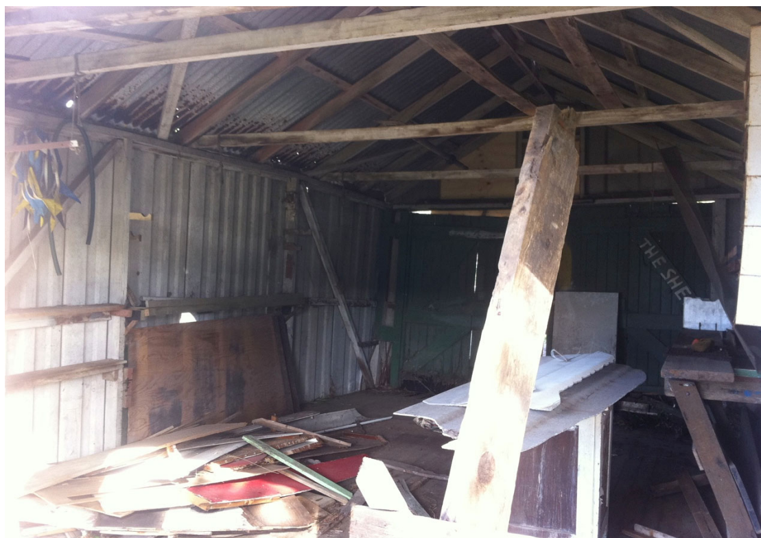
Internal view showing holes in walls and roof, also collapsed floor toward the back
