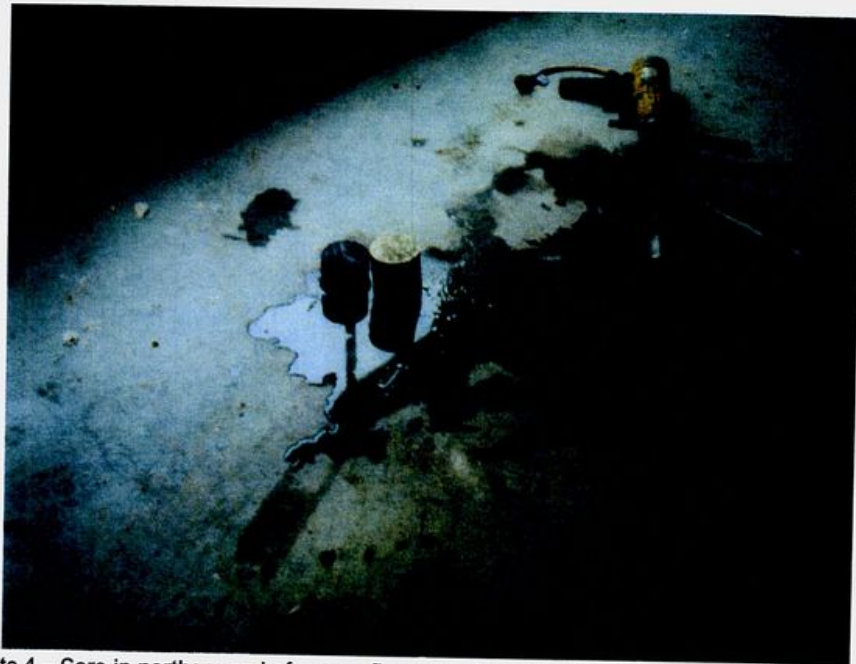
Photo 4 – Core in northern end of garage floor showing unreinforced topping, vinyl floor covering and original slab.
