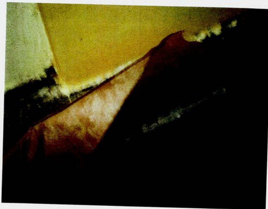
Photo 6 - Slab edge of eastern wall near window to dining showing the slab edge 110 mm in thickness overlying 1 course of bricks overlying original slab 90 mm in thickness
