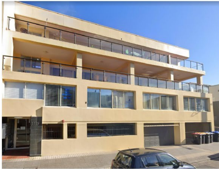
Figure 4: View of adjoining 4 storey mixed use development at No. 1119 Pittwater Road
