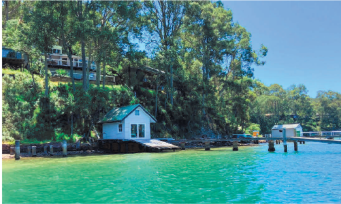
Photo 2: View from the Pittwater waterway of neighbouring Boat Sheds, i.e. No. 19 and No. 20 Portions.
