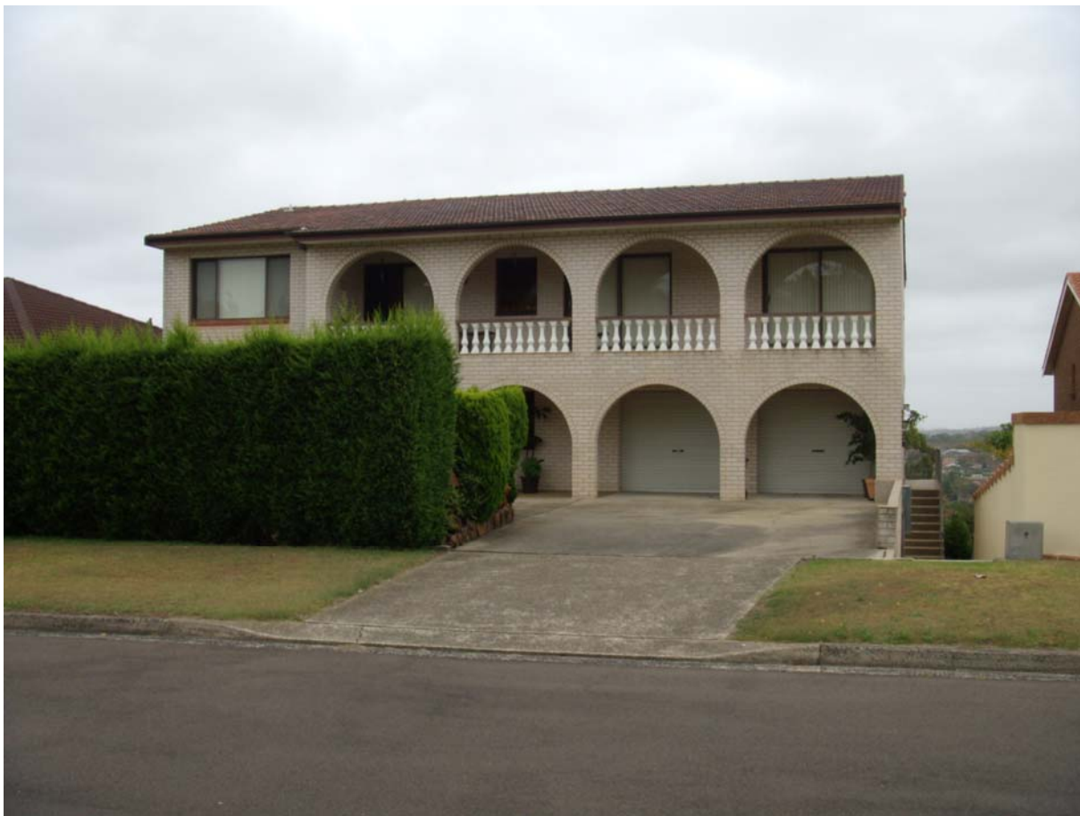
Photo 1: Subject site – No. 61 Lincoln Avenue, Collaroy
