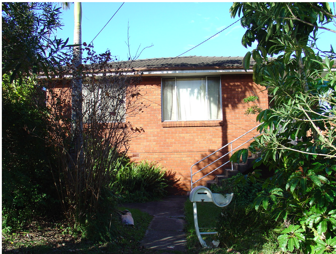
View of 1 Alfred Road from Alfred Road
