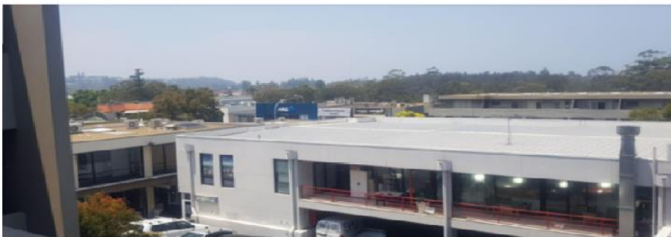
Image 8: Standing view from level 2 balcony looking north-east.
