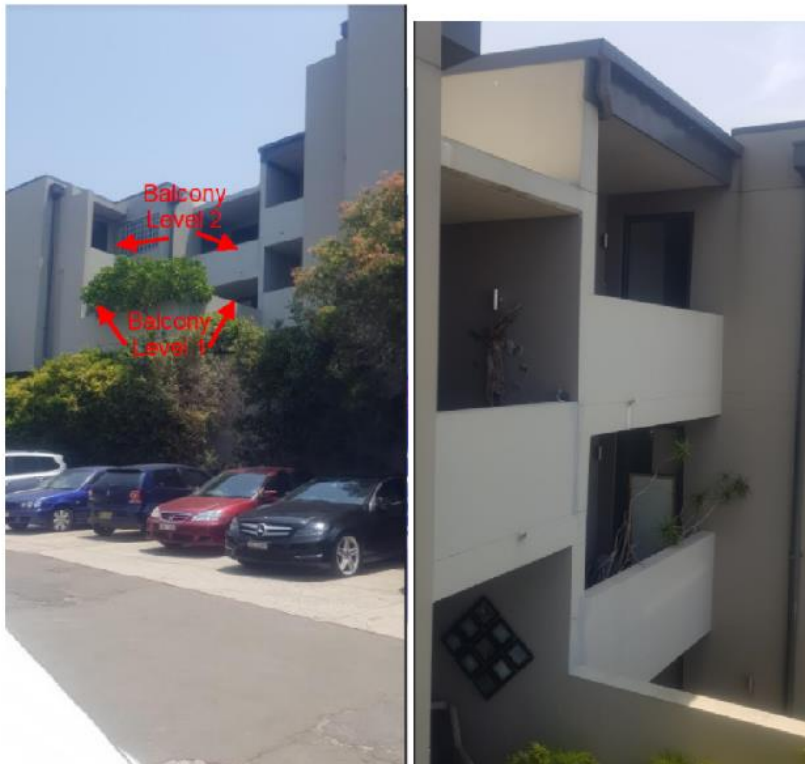
Image 1: Rear elevation of 24 Waratah Street showing the balconies to level 1 and 2 where view loss has been assessed.
