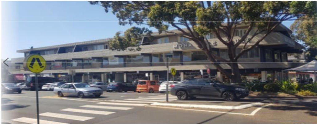
Three storey development to the east on the opposite side of Bungan Street.
