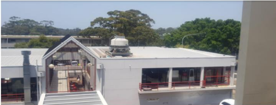
Image 7 : Standing view from level 2 balcony looking east.
