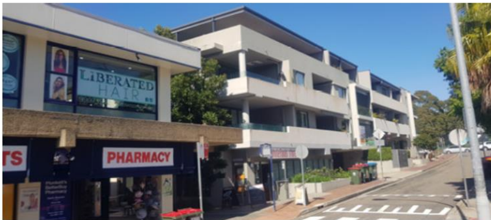
Three / four storey shop top housing to the west at 24 Waratah Street viewed from Akuna Lane.
