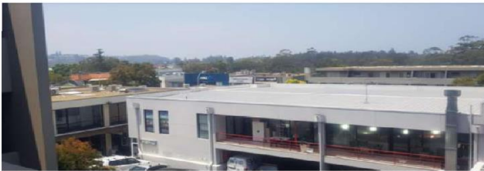
Image 8: Standing view from level 2 balcony looking north-east.
