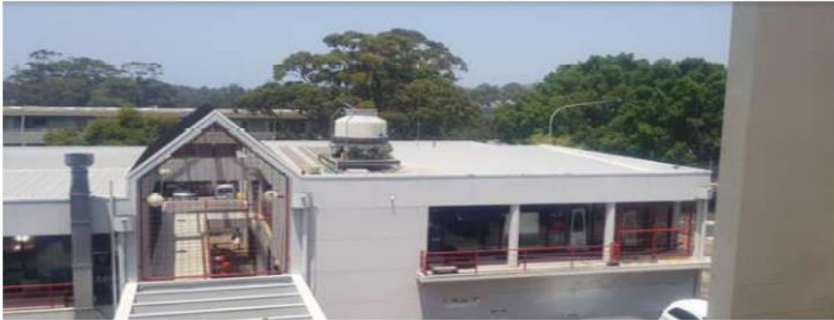
Image 7 : Standing view from level 2 balcony looking east.
