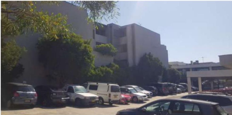
Three / four storey shop top housing to the west at 24 Waratah Street viewed from the subject site.
