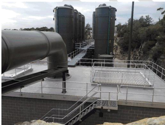
New bio-trickling filters at North Head WWTP
