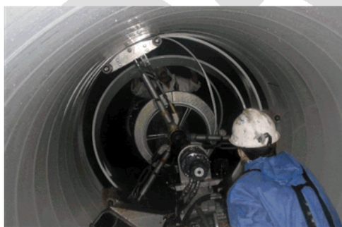
Installing the new structural liner
