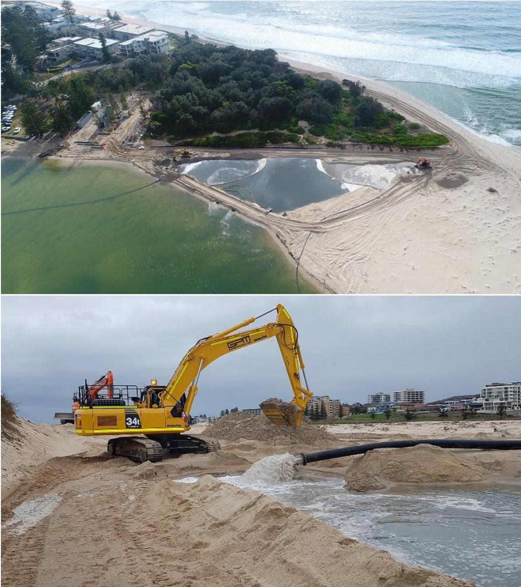
Figure 6-6: Management of sand slurry discharge within a bunded beach area at The Entrance, Central Coast
