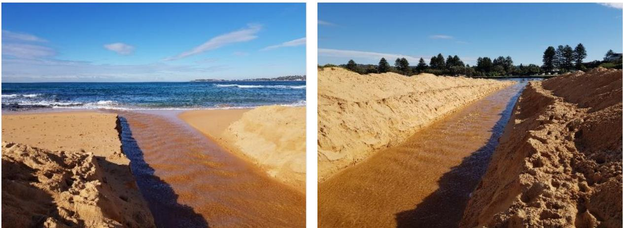
Figure 2-15: Mechanical opening of the lagoon entrance (4 June 2021)
