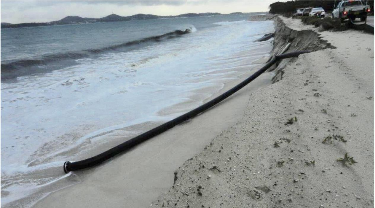
Figure 6-5: Damage to Jimmys Beach sand transfer system by large swell in 2019 (Source: Newcastle Herald, 5 June 2019)
