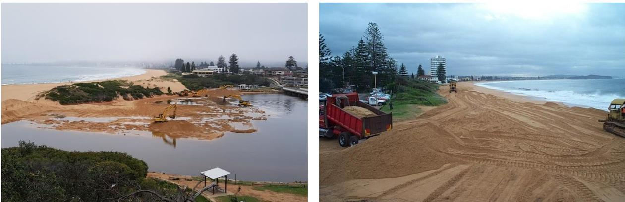
*Figure 5-1: Excavators removing the entrance shoals (left), Unloading and regrading of sand for beach replenishment (right)*
