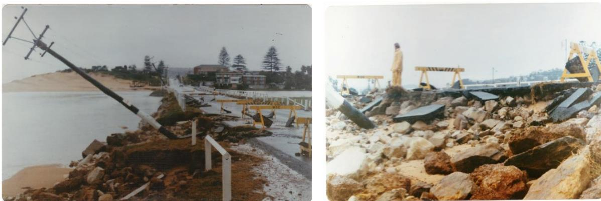
Figure 2-12: Damage to Ocean Street Bridge in 1974
