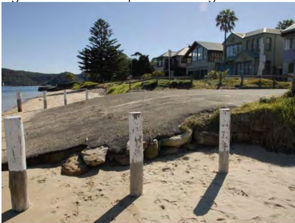
Figure 37. Erosion to edge of ramp.
