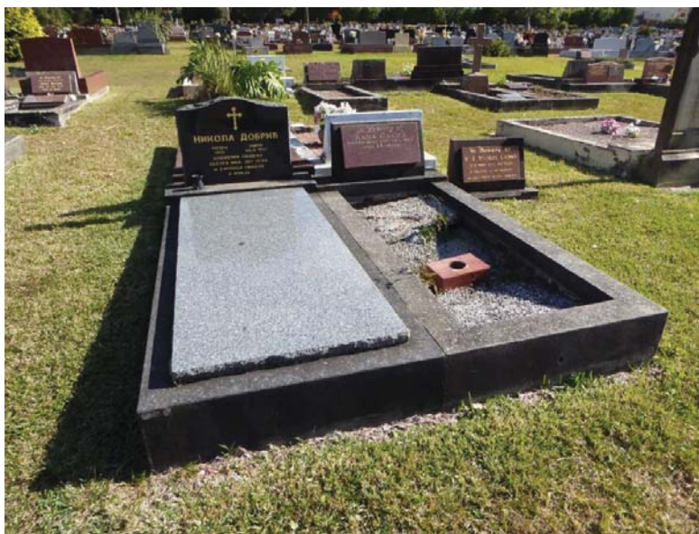
Figure 18 Pair of desk and slab type memorials. The original slab on the right-hand grave has failed, probably due to subsidence of the soil and remains below. The left-hand grave has a granite slab above the kerb, possibly added to hide a similar problem to the right-hand grave. (Photo: Chris Betteridge, 6 July 2016)
