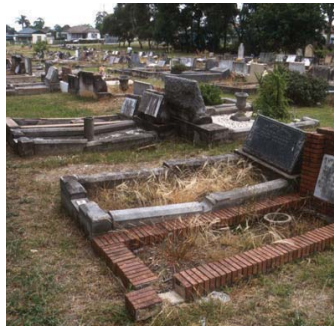
Coffin collapse can cause leaning headstones or broken kerbing
